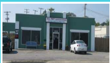
Our building houses more than just an adoption facility! We also have low cost vet services, behavioral consultations, and volunteer opportunities!
